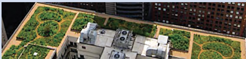
Figure: The green roof on top of Chicago's City Hall is designed to cool the building and increase energy efficiency. Image courtesy of City of Chicago ( http://www.chicagoclimataction.org/pages/research_reports/8.php ).
